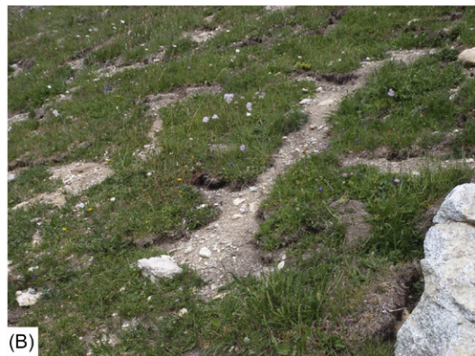
FIGURE 8.49 (A) Advanced filling construction with direct-shifted sods integrating structural elements such as boulders and dwarf shrubs. The sods and their root horizons are removed from behind the excavator as the filling gains height. (B) Sod mosaic with irregular gaps 1 year after direct-shifting. Before the emergence of complete vegetation cover through the expansion of the autochthonous flora, small-scale erosion and accumulation of soil material within the gaps may occur. These processes can be accepted as they contribute to site-specific heterogeneity. Source: photos: N. v. Albertini.
